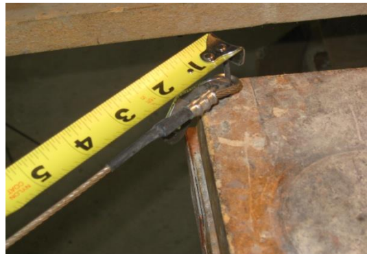
Figure 12 - Cable Measuring Fixture
