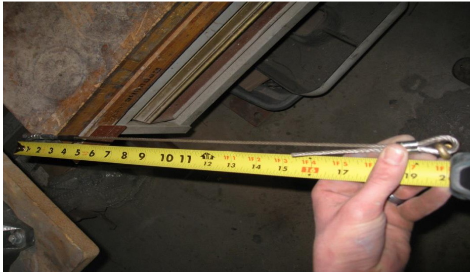
Figure 13 - Measuring Cable to Length
