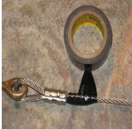
Figure 16 - Chafe Tape Installation
