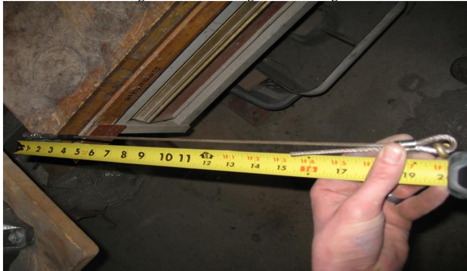
Figure 14 - Measuring Cable to Length
