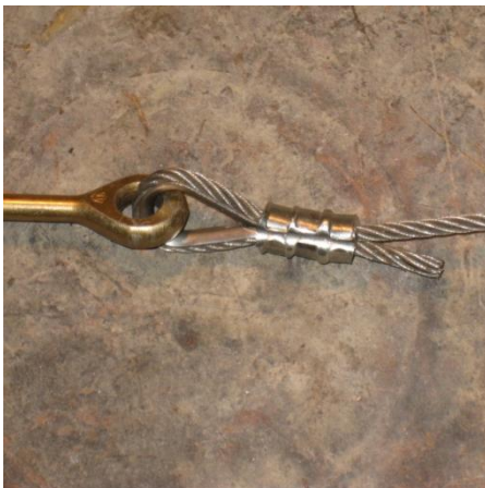
Figure 15 - Cable Finished to Length
